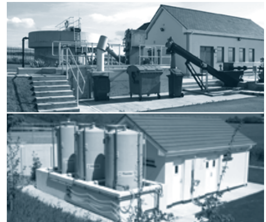
sample projects completed: ballyheigue sewerage scheme and mogeely water supply scheme
